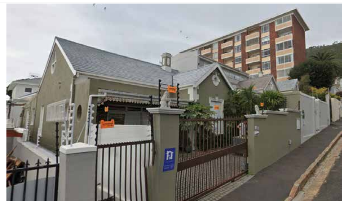
Heathfield Road Grade 3C
