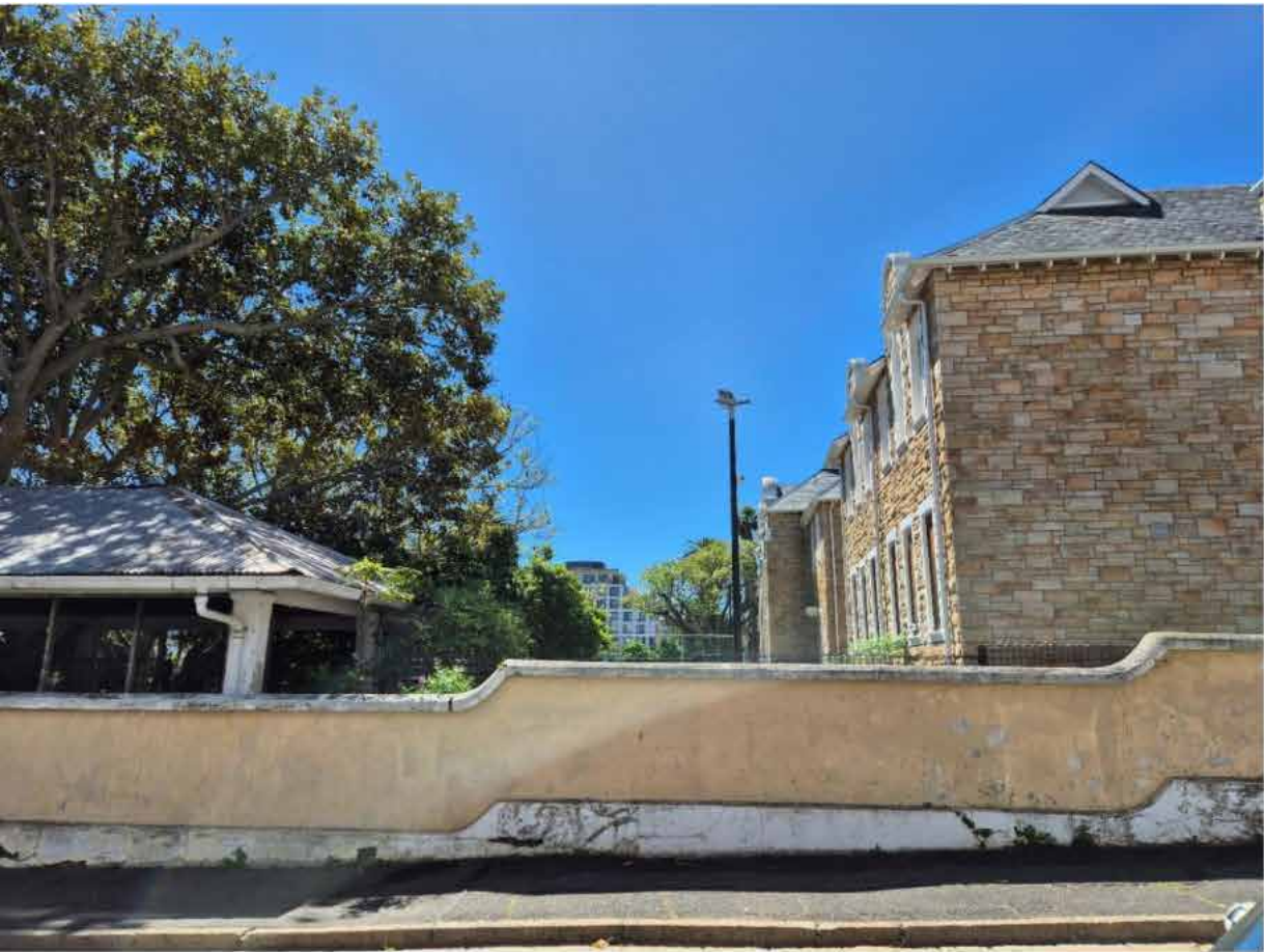
Figure 110. Viewpoint 2, looking northeast from The Glen towards the Portion 1 development site (Square One, 2025)
