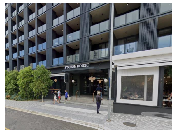
Figure 2-5 Active ground floor with residential units above. (19 Kloof Road, Sea Point).
