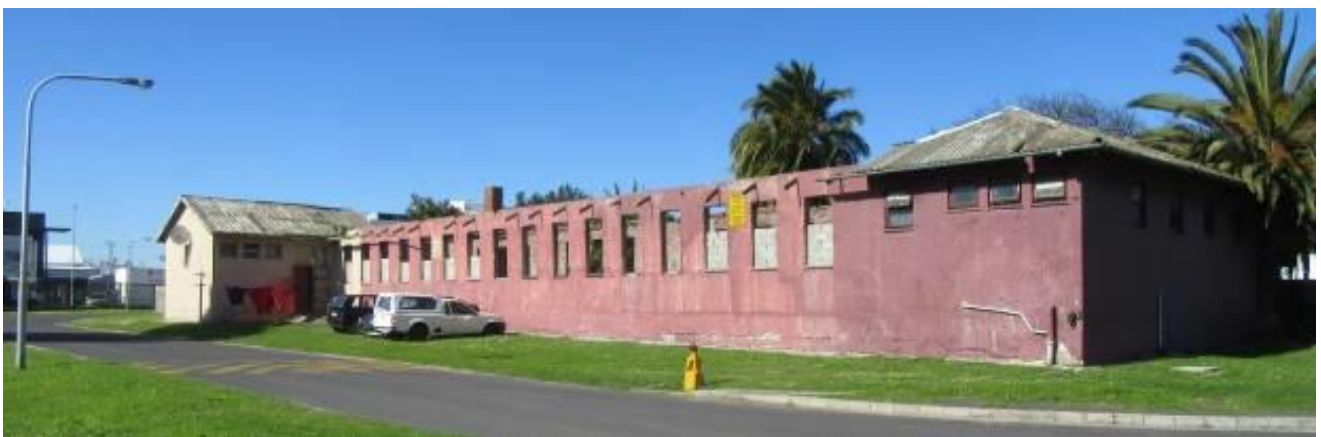
Photograph 4.9: North-facing portion of Block B which was destroyed by fire sometime late 2000 or early 2001. Block B mainly accommodates residential uses.
