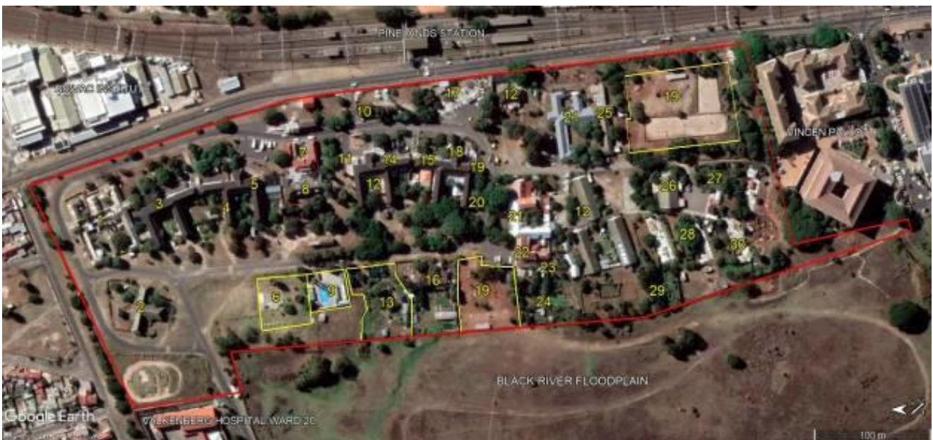
Figure 4.1: Key tenants, land uses and designated use areas (yellow outlines) on OMV site (red outline) referred to in report.
