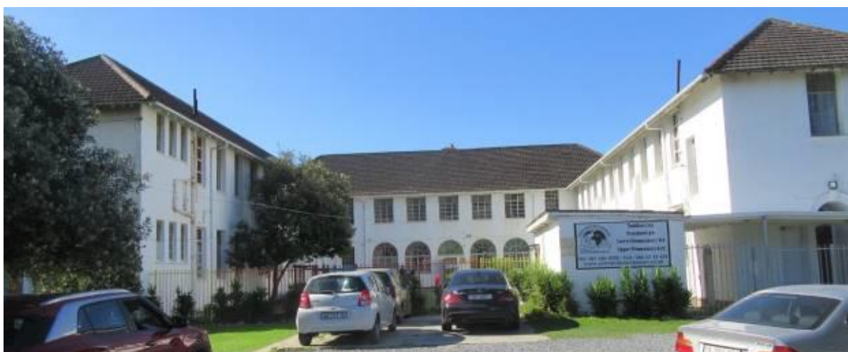
Photograph 4.4: Pinelands Montessori School, Block C.
