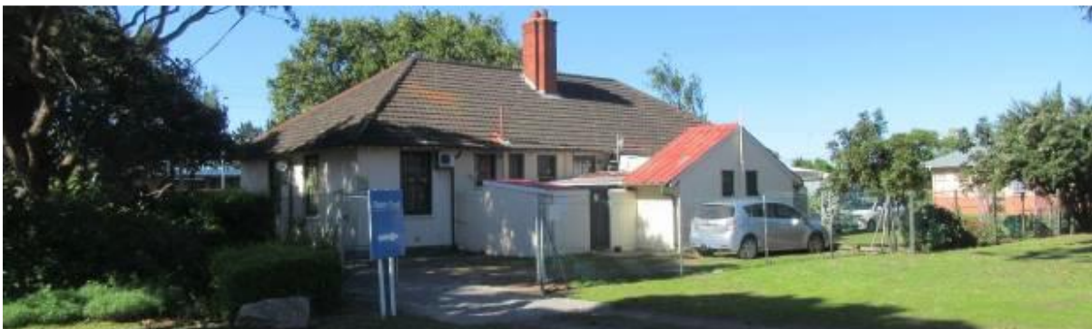
Photograph 4.7: Robin Trust, administrative building (Block R).
