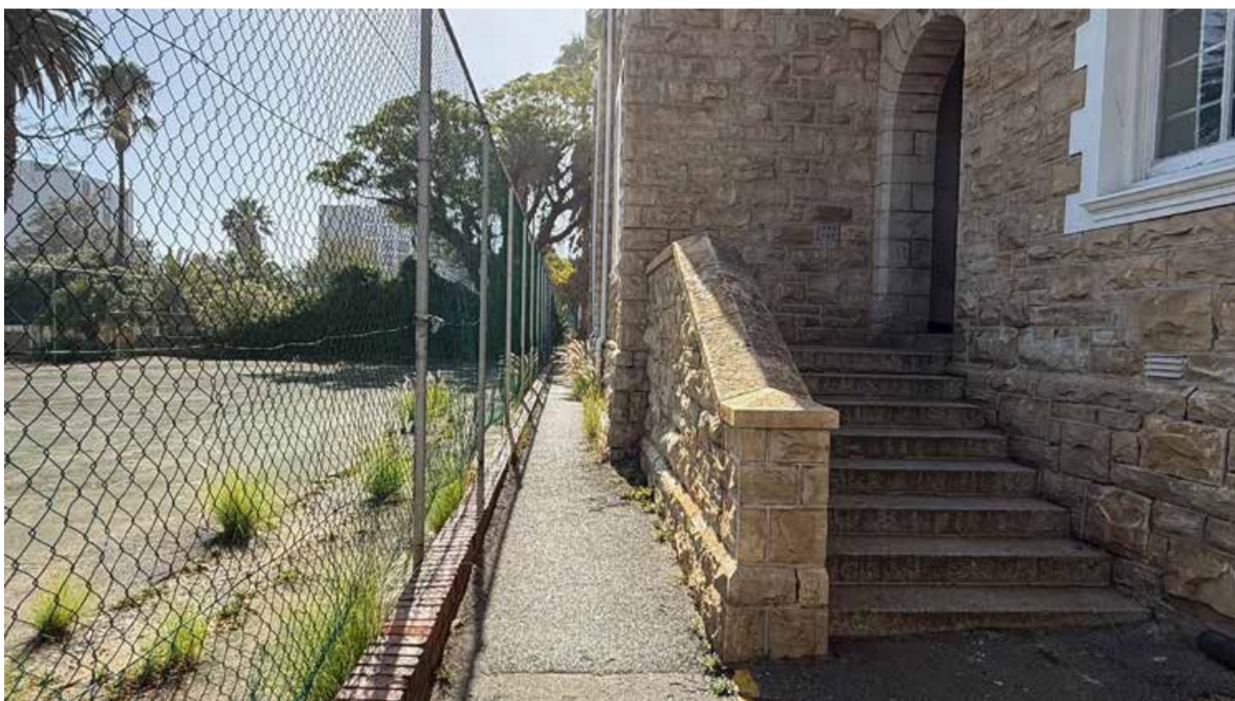
Current front facade of school and garden interface
