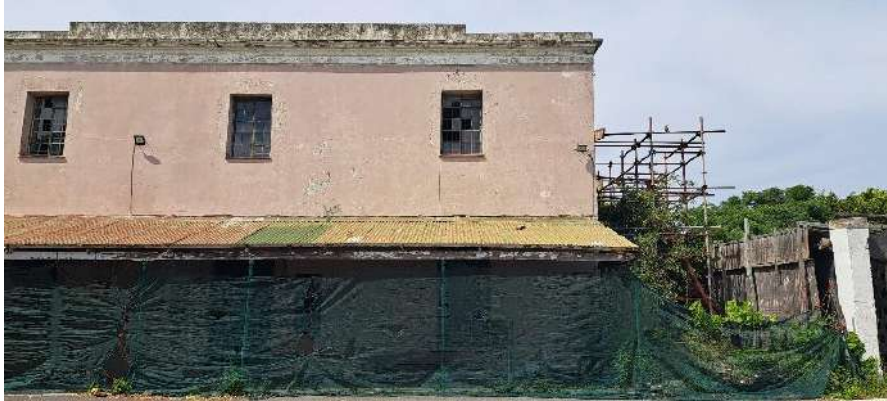
Figure 94: Condition of the Homestead (November 2023)
