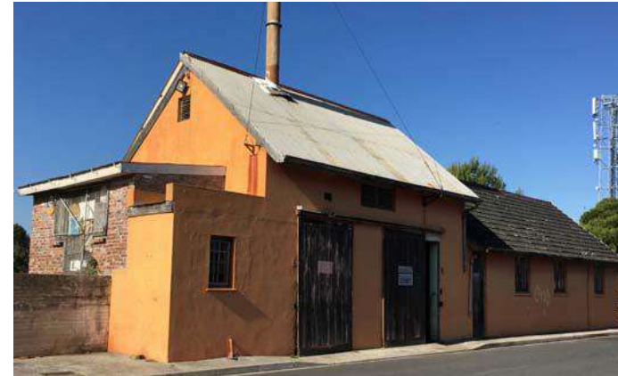
Block Q staff house: Fair condition; leaking roof and wall cracks. Retain and upgrade with minimal fabric intervention.
