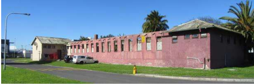
Figure 73: North-facing portion of Block B which was destroyed by fire sometime late 2000 or early 2001. Block B mainly accommodates residential uses.
