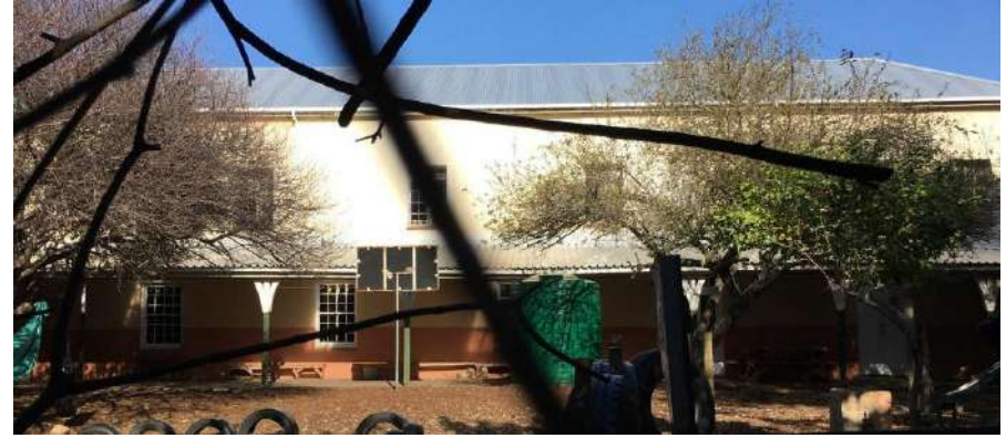
Figure 96: Front/north elevation of early 20th century addition (Wilson 2022)
