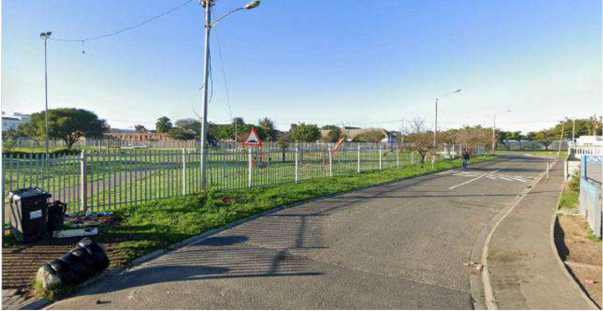
Figure 180: View C: Southwards from Maitland Garden Village, across existing Green Open Space.
