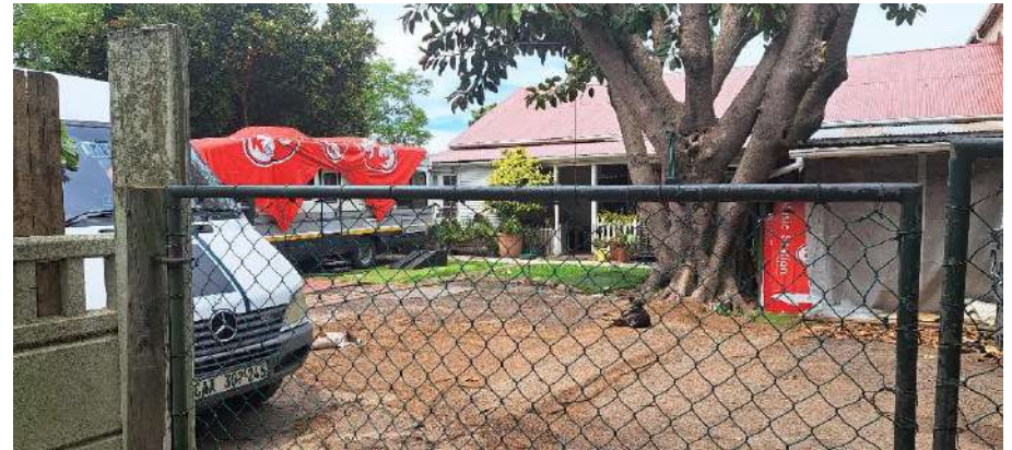
Figure 97: Victorian cottage attached to the early 20thC addition (Block W)
