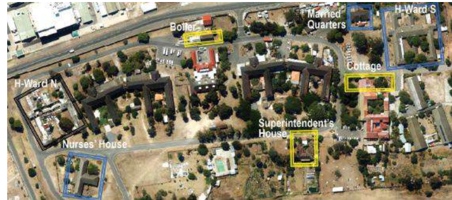
Figure 133: Aerial view of the Boiler, Nurses House, Superintendent's House, Cottage, Married Quarters and the H Wards, Winter, Baumann & Wilson 2022
