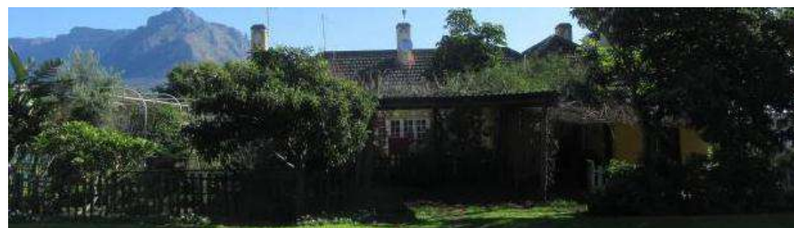
Figure 71: 'The Yellow House', used by residents as a demonstration model of various sustainable resource use practices.
