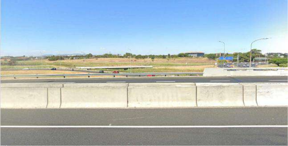
Figure 174: View E: Eastwards from the M5 bridge over the N2 across the Black River
