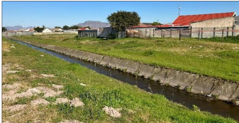
Figure 6: Canalised section of the Big Lotus River west of the site (Liz Day Consulting, 2025)
