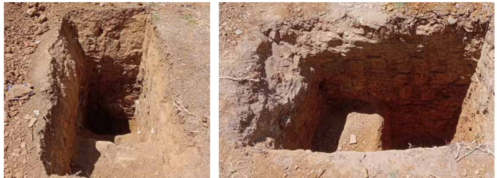
Figure 22. Test Pit 3 (right) and Test Pit 4 (left) (RSA, 2025a)
