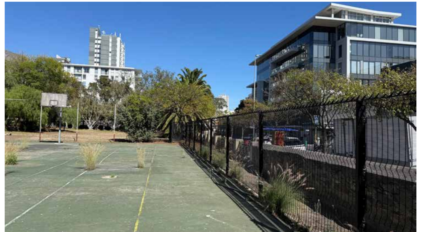
Figure 194. The DSD site should be kept weed free and tidy and a tree and landscaping maintenance plan put in place (RSA, April 2026)
