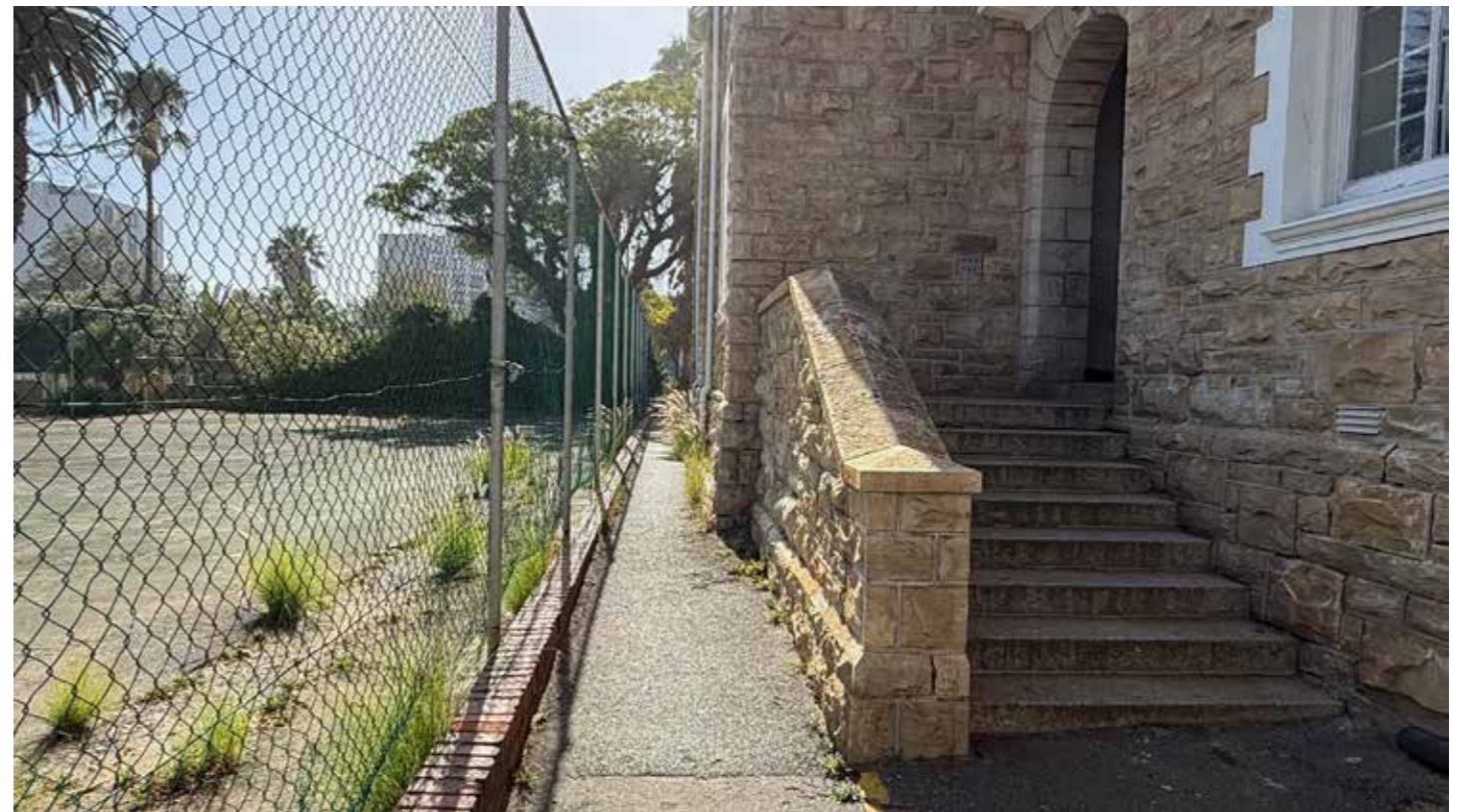
Figure 89. The present interface condition between the front façade of the school and the fenced in tennis court is not positive and a more open landscaped interface condition and integration of required parking can be facilitated here (RSA, April 2026)
