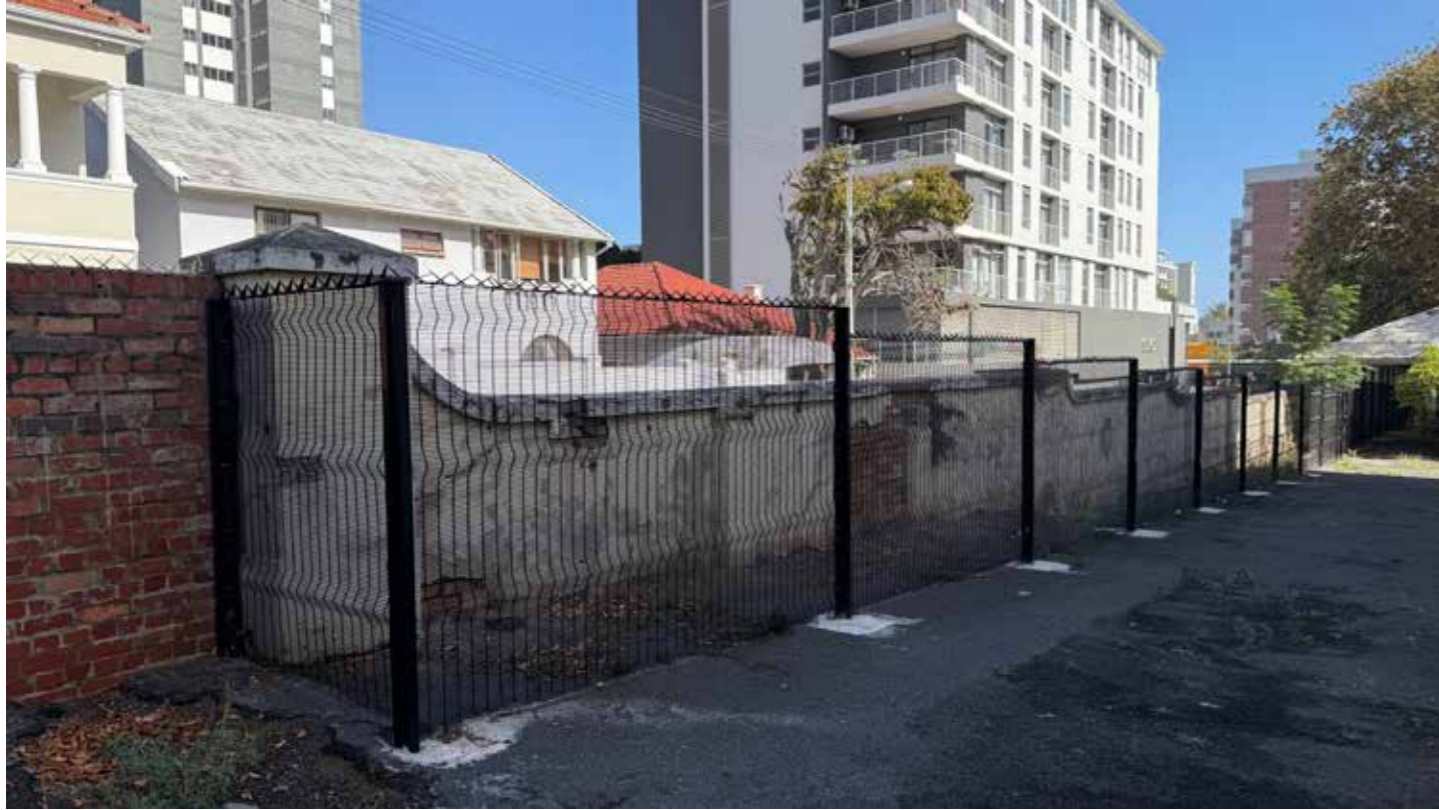
Figure 175. Careful conservation work using appropriate lime mortars and renders to historic boundary walls to be undertaken. Areas of hard cement, plaster and inappropriate coatings to be removed (RSA, April 2026)
