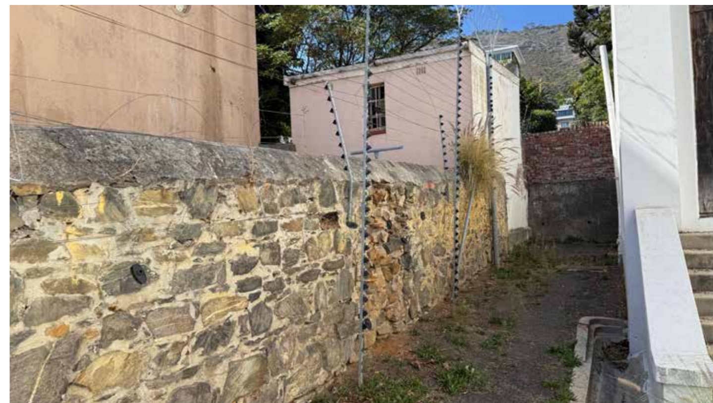
Figure 93. View of the historic stone walling to be retained and incorporated in the pedestrian walkway and junction with Herbert Road. (RSA, April 2026)
