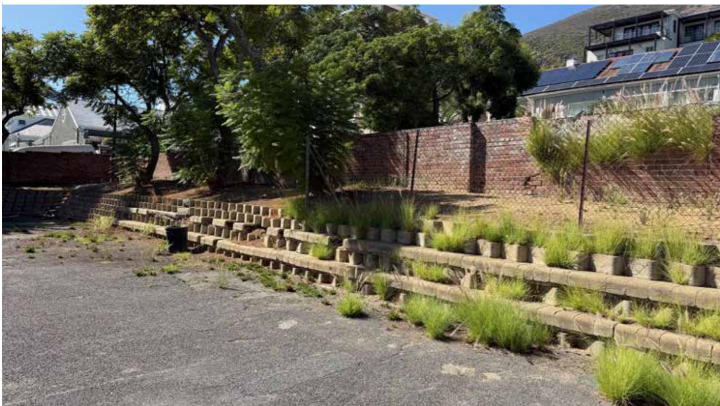
Figure 196. A general site review of low walls, terracing, fencing etc is required to ensure that the property does not degrade (RSA, April 2026)
