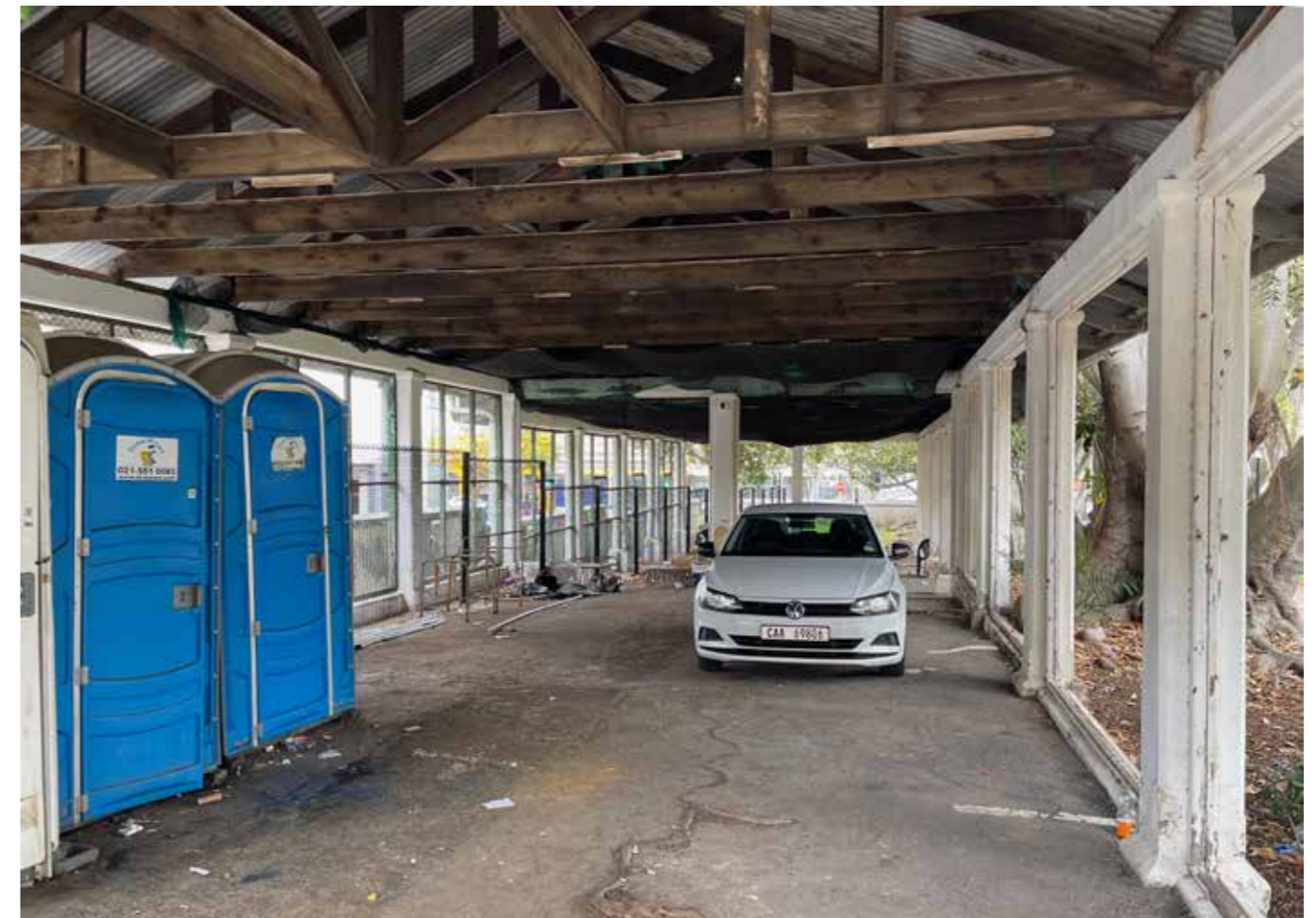
Figure 76. Bike shed, with a vehicle to demonstrate scale. (RSA, 2023)
