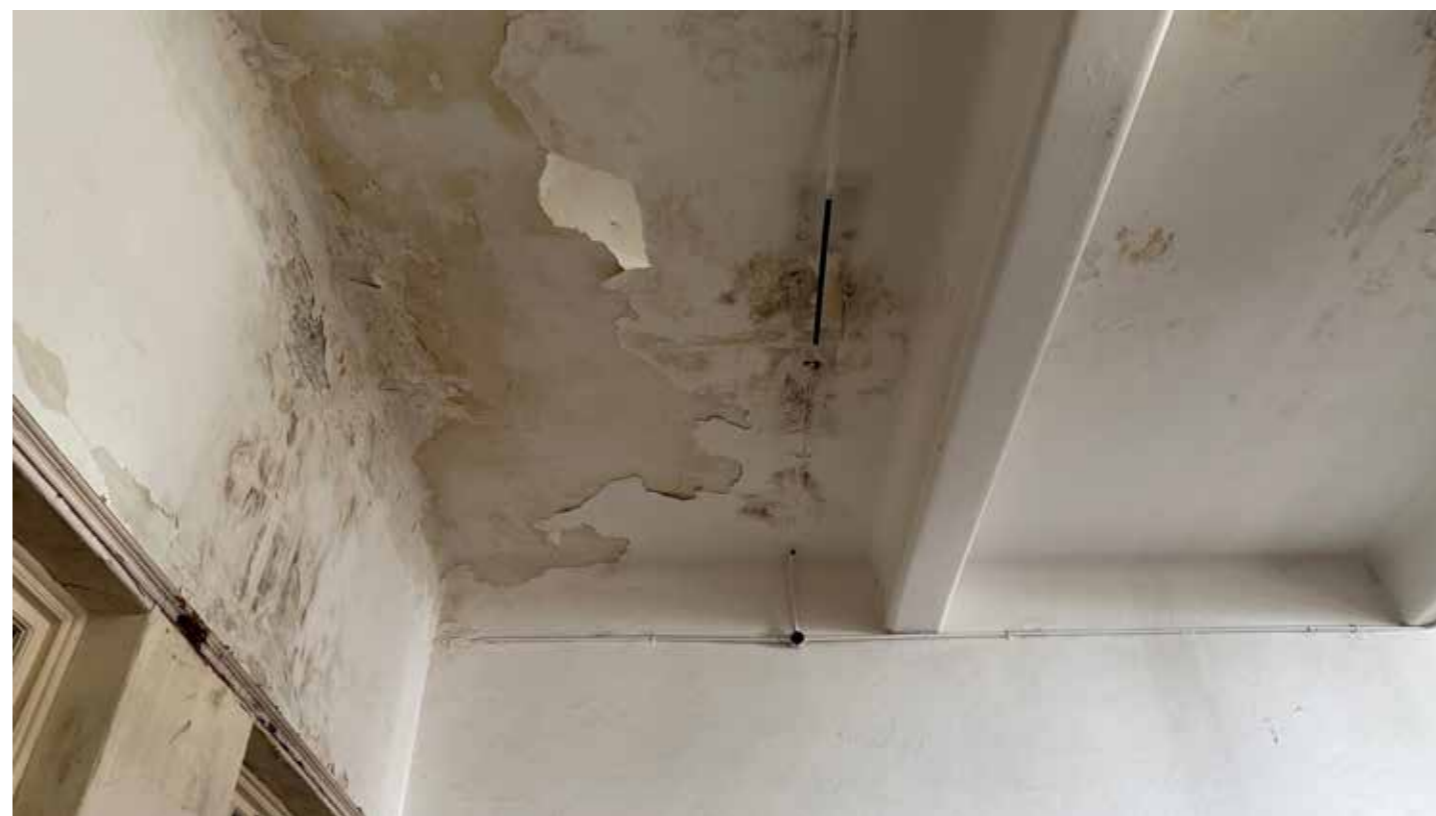
Figure 182. Ensuring that the building remains watertight is an essential component of any maintenance plan (RSA, April 2026)
